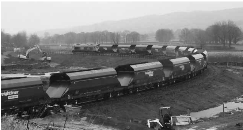
Above Right: The sidings completed. Below: The test train reverses in through the rain. Photos: Mike Farrington
