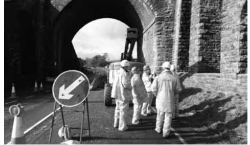
At the bridge over the A684 just beyond Moorcock Viaduct
