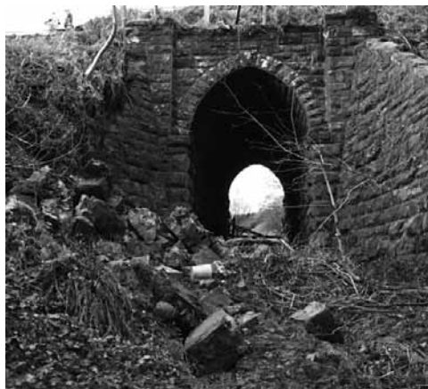
Wing wall collapse at Bridge 323
