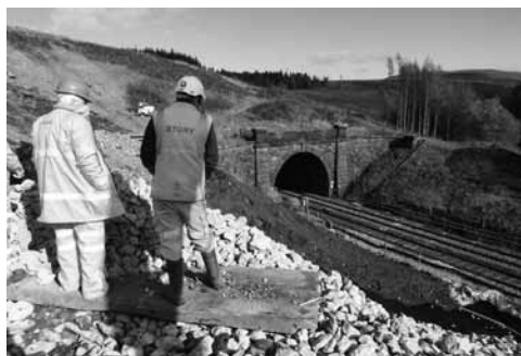
Looking towards the south portal of Rise Hill tunnel
